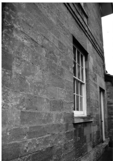
Figure 24 Evidence of former doorcase on east wall in 'catrun'
