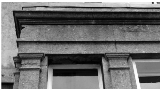
Figure 22 Stone pilasters on west front of crosswing
