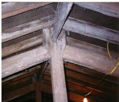
Figure 12 King post roof in north section
