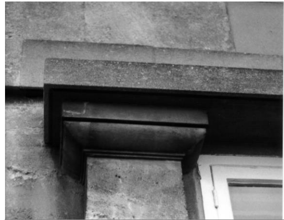
Figure 20 Stone lintel on west front of northern section
