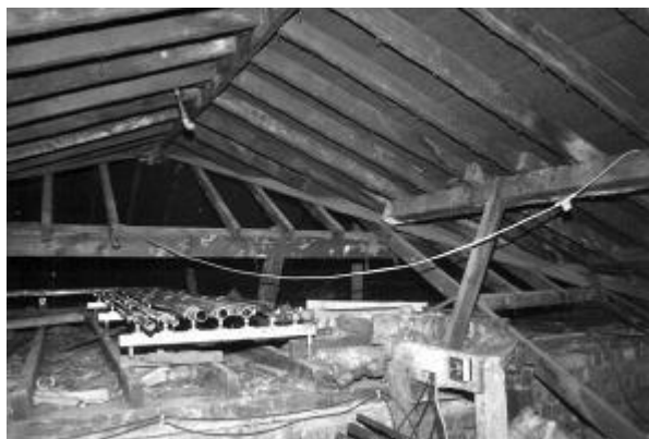
Figure 11 Interior of roof looking north
