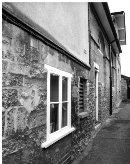
Figure 10 Stonework in 'catrun' on east wall
