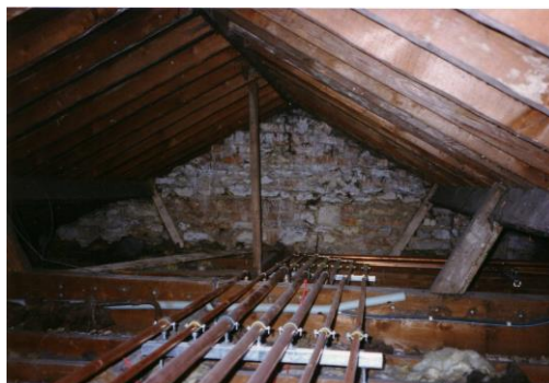
Figure 13 Interior of southern crossing
