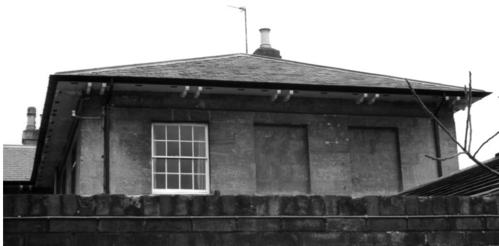
Figure 17 Double modillions in northern section of house
